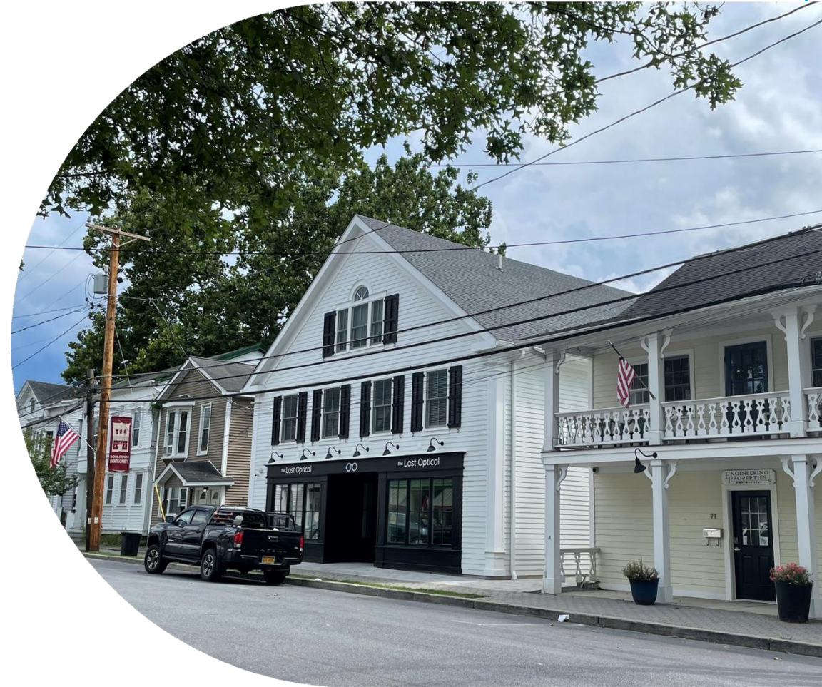
INFILL DEVELOPMENT, MONTGOMERY, NY
